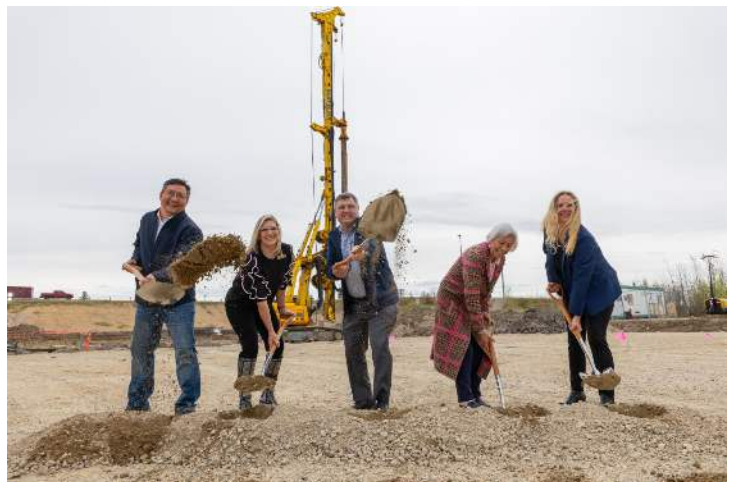
CASA Mental Health and Government of Alberta officials celebrate the start of construction on CASA House Fort McMurray on May 22, 2026. Photo credit: Nicholas Vardy
